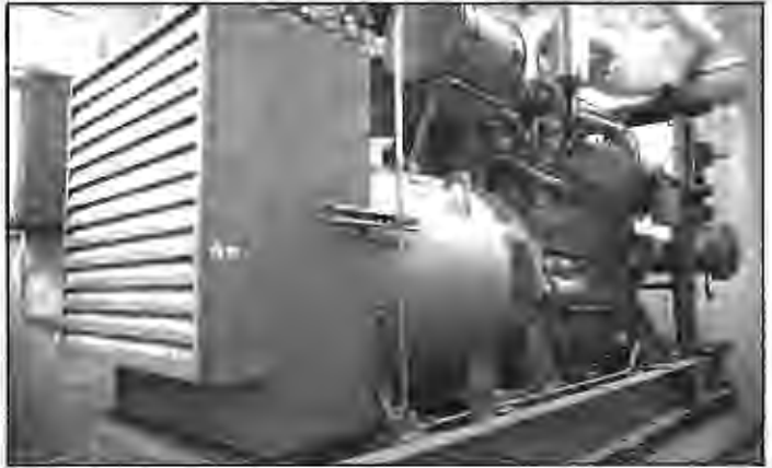
At the bottom of it all: a 450 kw emergency generator capable of keeping the ABC Washington news operation on the air for one week.
